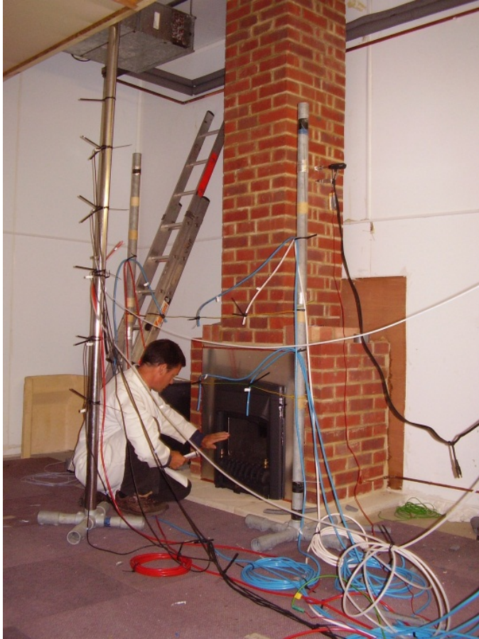
Figure 3 Purpose - design fireplace and test chimney
